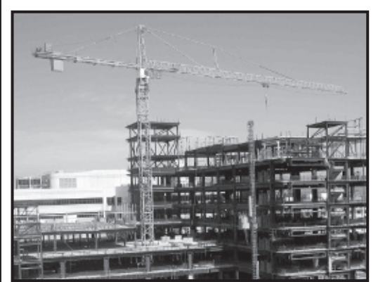
CHOC's new state-of-the-art tower will change Orange County's skyline. Pictured is the 200-foot-tall crane, visible from across the city, which will be removed from the construction site this month.
